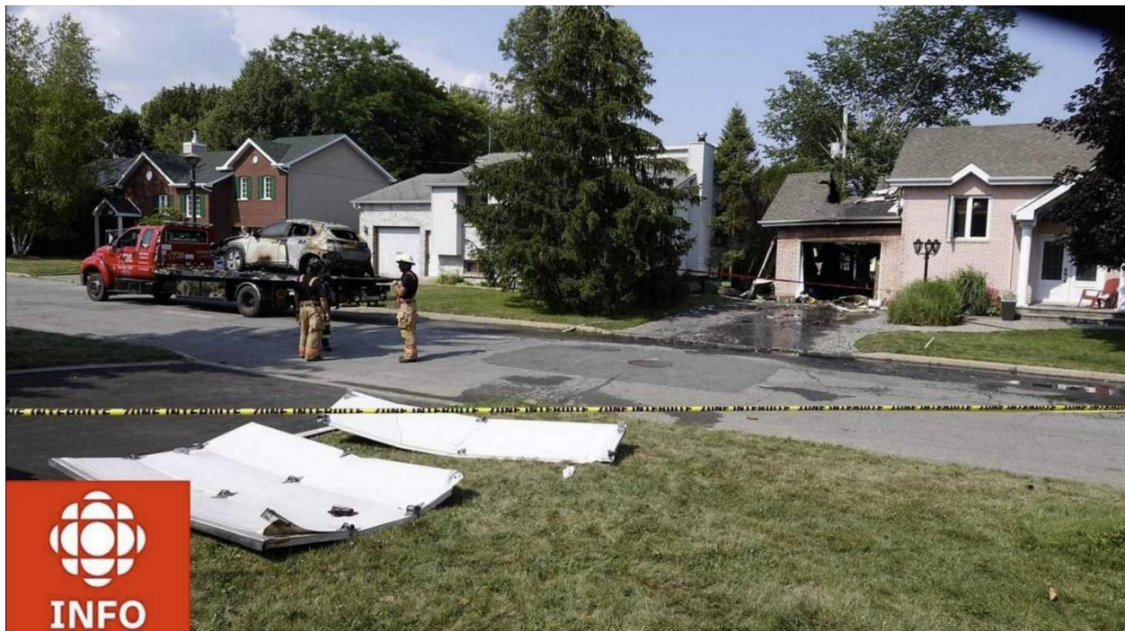
Figure 12 – Garage condition following incident [19].
