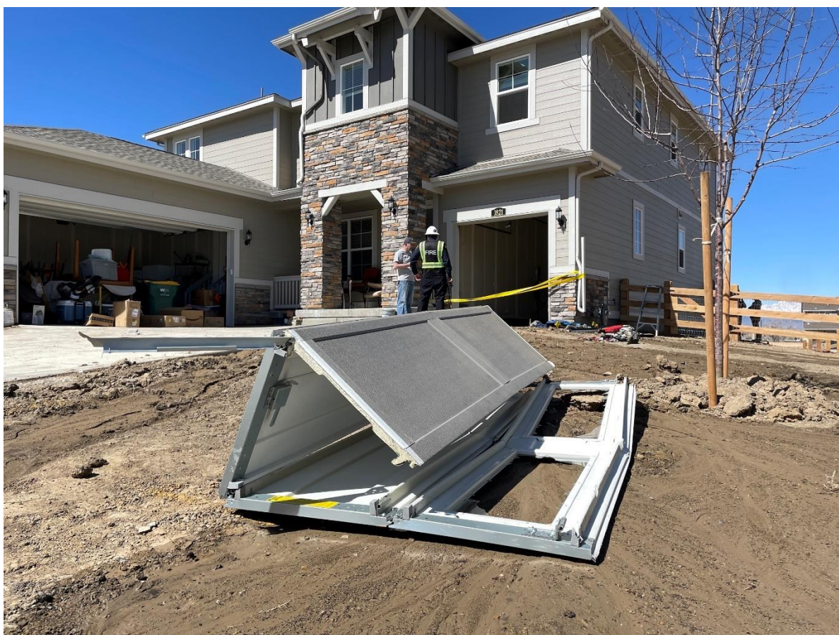
Figure 21 – Garage door location following garage explosion [26].
